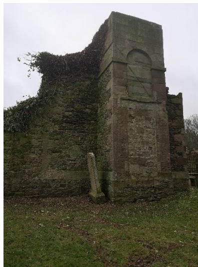
At last, we can see the top of the bell tower
