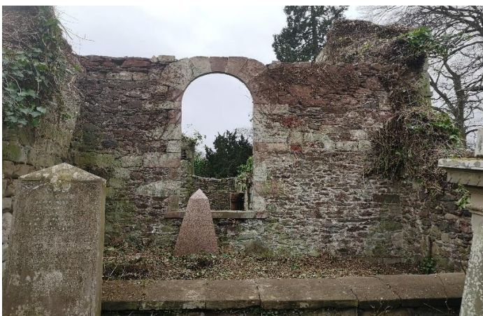
The Skene burial aisle with the arched window in the east wall of the north transept
