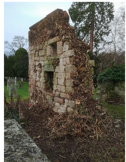
Part of the south wall with two windows visible
